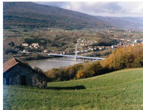
The Seyssel Bridge over the River Rhone
