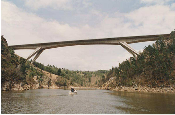
The Truyère Viaduct on the A75 Motorway
