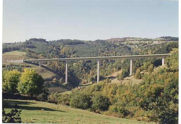
The Piou Viaduct on the A75 Motorway
