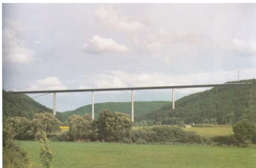
The Neckar Viaduct at Weitingen (1977)
