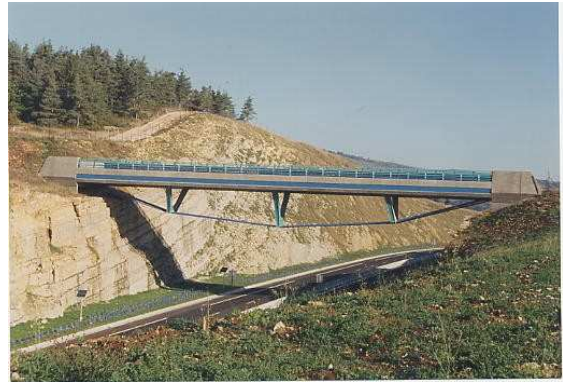
The Truc de la Fare overpass on the A75 Motorway
