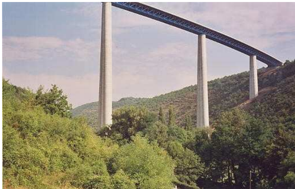
The Verrières Viaduct on the A75 Motorway
