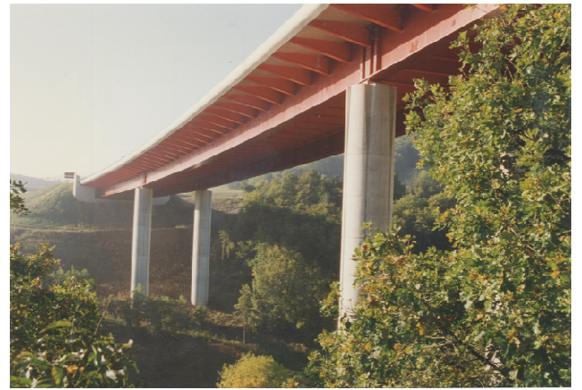
The La Planchette Viaduct on the A75 Motorway
