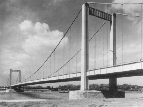
The Cologne – Rodenkirchen Bridge (1938)
